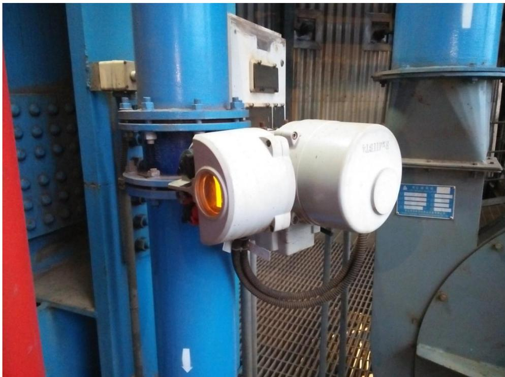
Gambar : 2.25 MOV outlet duct burner fan
