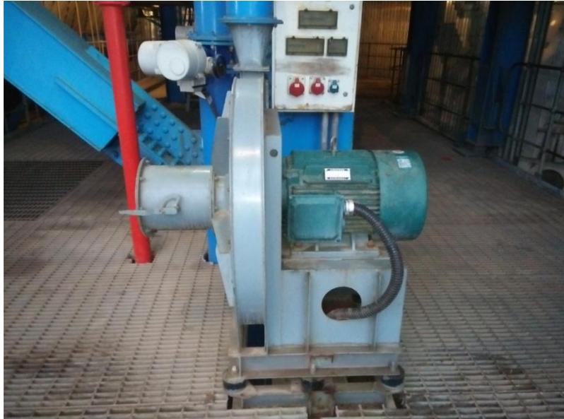
Gambar : 2.23 *Duct burner fan*
