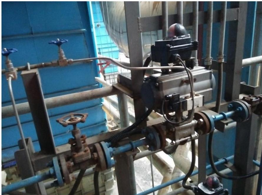
Gambar : 2.21 *Manual dan pneumatic valve purging duct burner*
