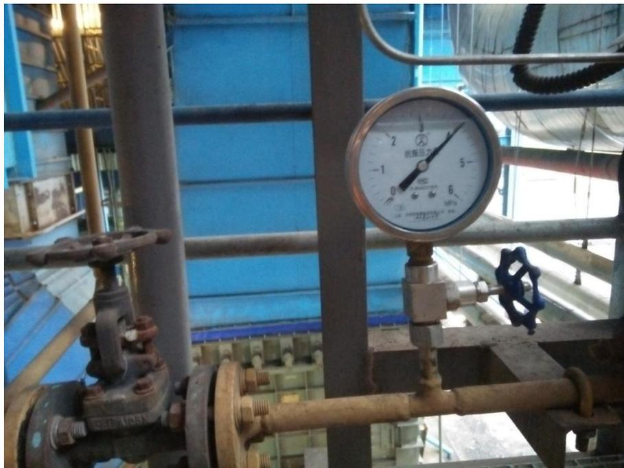
Gambar : 2.19 *Pressure gauge supply HSD ke duct burner*
