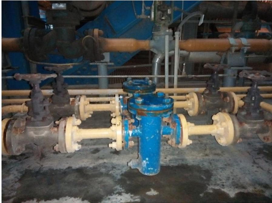
Gambar : 2.10 *Filter supply return HSD tiny oil*
