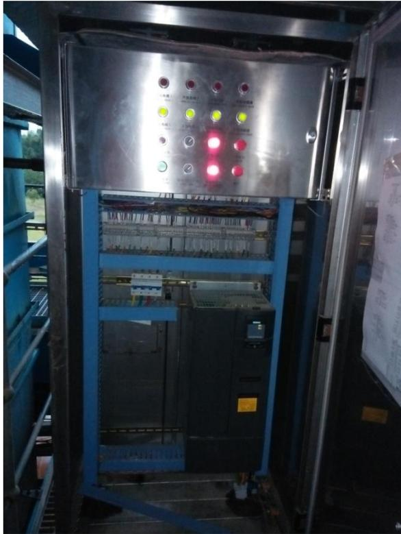
Gambar : 2.24 Kontrol panel lokal *duct burner*
