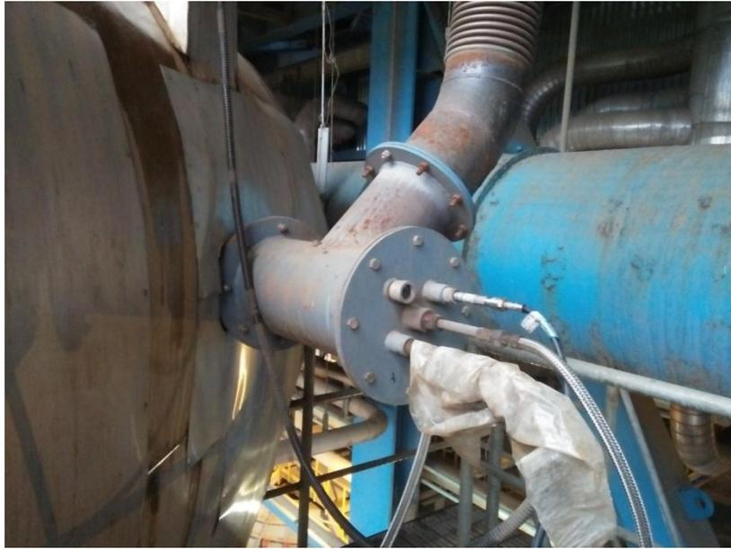
Gambar : 2.19 *Duct Burner*
