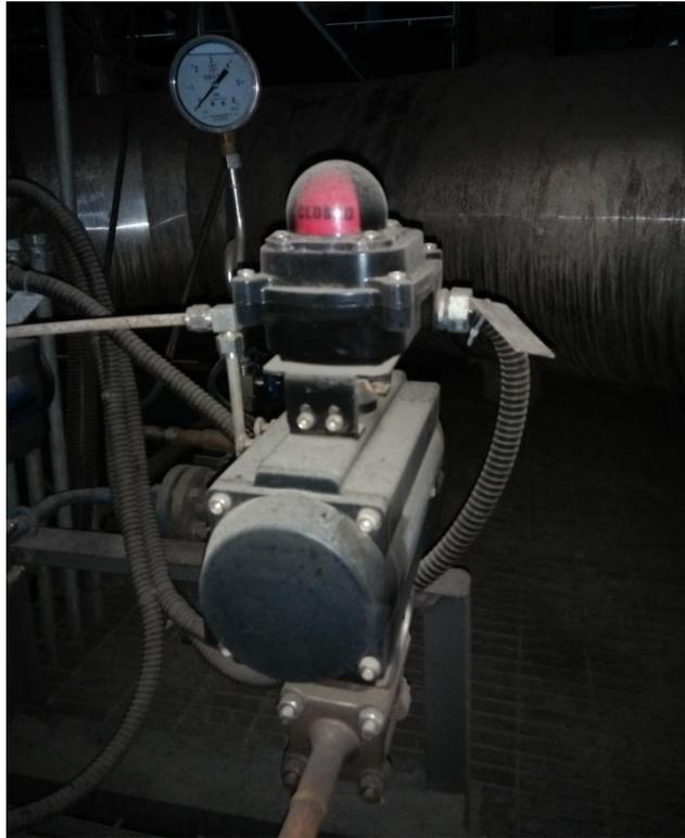
Gambar : 2.14 *Pneumatic valve suply tiny oil*
