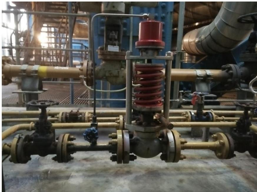
Gambar : 2.9 *Pneumatik valve main supply tiny oil*
