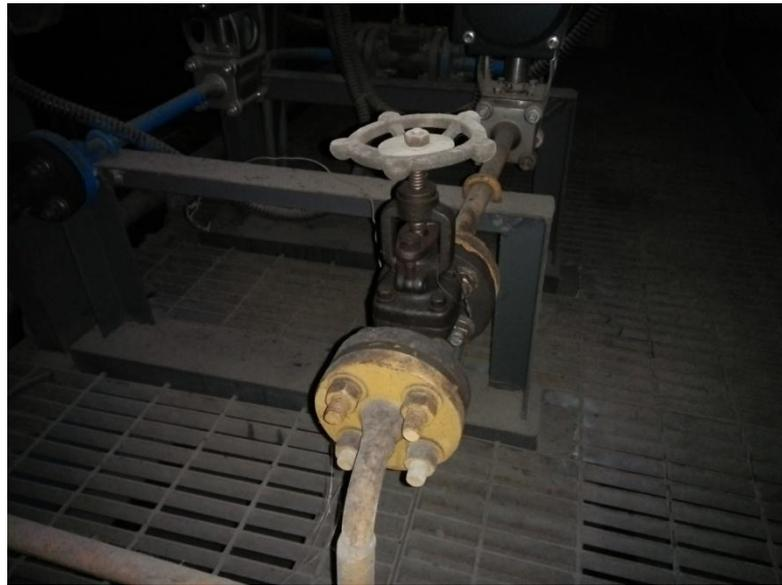
Gambar : 2.17 *Manual valve supply tiny oil*
