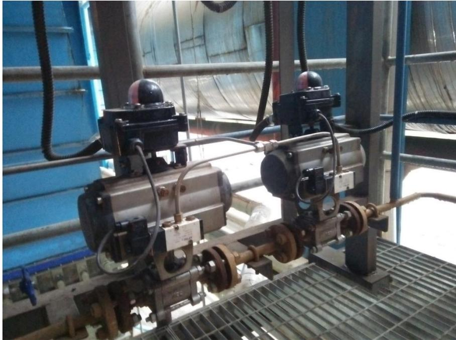
Gambar : 2.22 *Pneumatic valve supply HSD duct burner*
