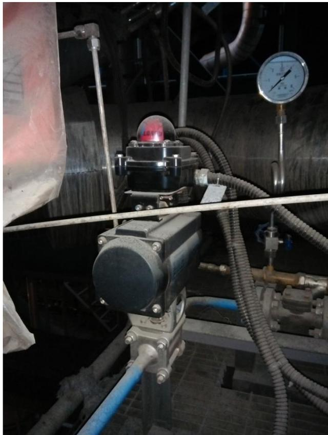
Gambar : 2.15 *Pneumatic valve purging tiny oil*
