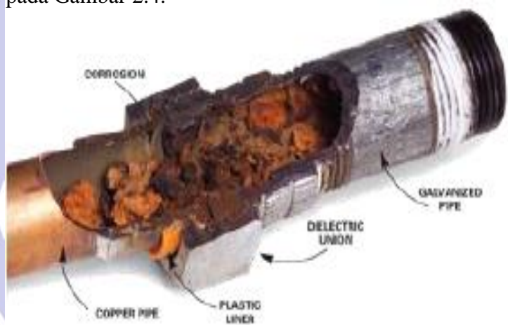
Gambar 2.4 Korosi Galvanik ( Corrosionclinic , 2013)
