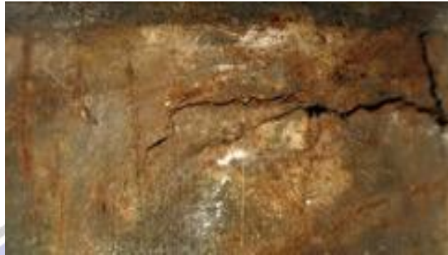
Gambar 2.5 Korosi Sumuran ( Scribd.com/korosi )
